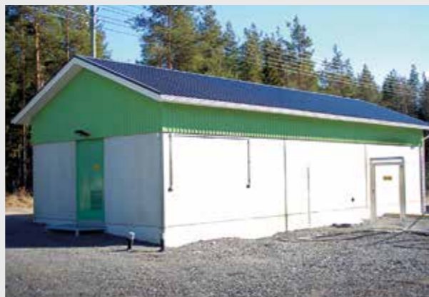
Concrete-framed fire class P1 equipment shelter.
